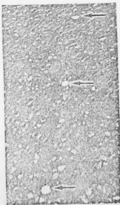
Tricolored discs like this are cemented into the pavement (see below, arrowed). Wear is measured by visual examination of the color which shows
