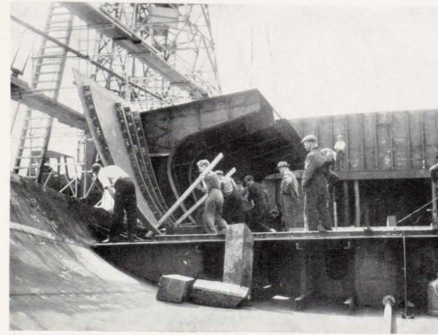
TWO STAGES IN THE CONSTRUCTION OF A PREFABRICATED TRAWLER: Left—A section of deck and hatch girder is secured in place in the yard of Brooke Marine, of Lowestoft. Right—The bow section is fitted to an Arctic trawler, one of the order for twenty for the Soviet Union which this firm of shipbuilders and engineers is building in its yard on the Suffolk coast.
