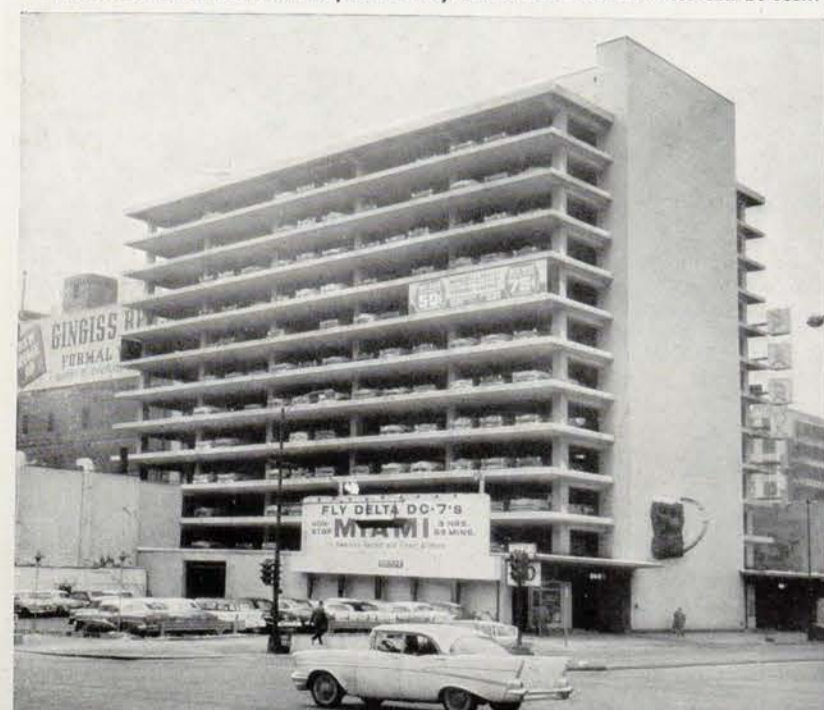
A MODERN PARKING LOT: "World's largest mechanical parking garage" says the sign on this city-owned building on Wacker Drive at State Street, Chicago. A car can be left here all day for 3s. 6d. On right—Morning rush-hour traffic pours into Los Angeles off the Pasadena Freeway. Even the most modern highways are overloaded by the ever-increasing number of cars on the road.
