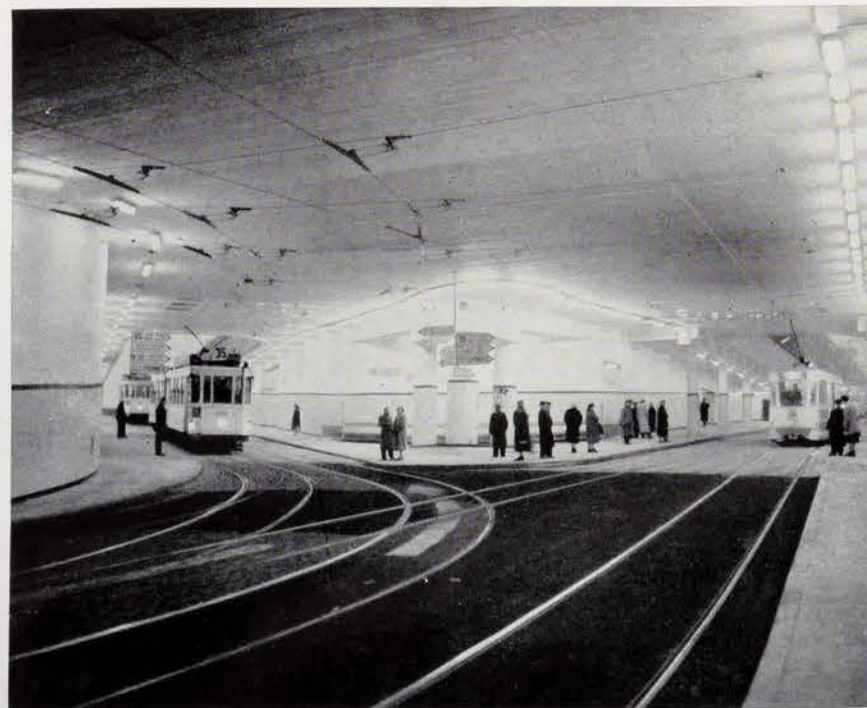
THE TRAM STATION BELOW THE CENTRE OF BRUSSELS: The platforms of the Carrefour Midi are beside a Y-shaped formation of lines. Until the completion of this underground system the trams were a main cause of traffic blocks above ground.
