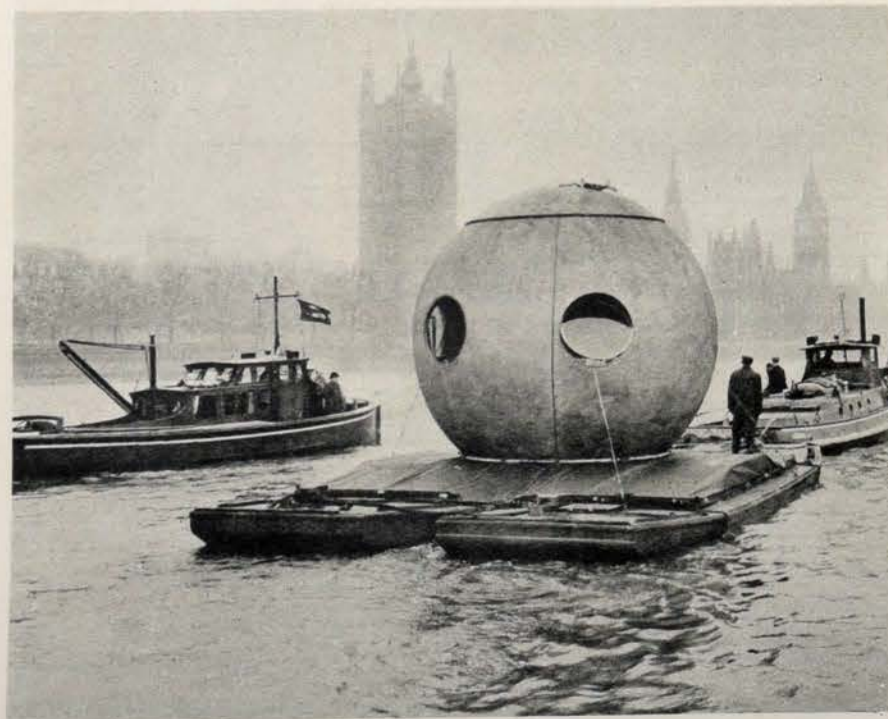
THE LAST WORD IN PREFABRICATION: The aluminium Round House, which will be on view at the Ideal Home Exhibition, is being towed up the Thames past the Houses of Parliament on its journey from Germany to Olympia. It had arrived in England in the hold of a freighter. At Chiswick it was put on a lorry and driven to Olympia. About 15 ft. in height and 13 ft. in diameter, it can accommodate two people.
