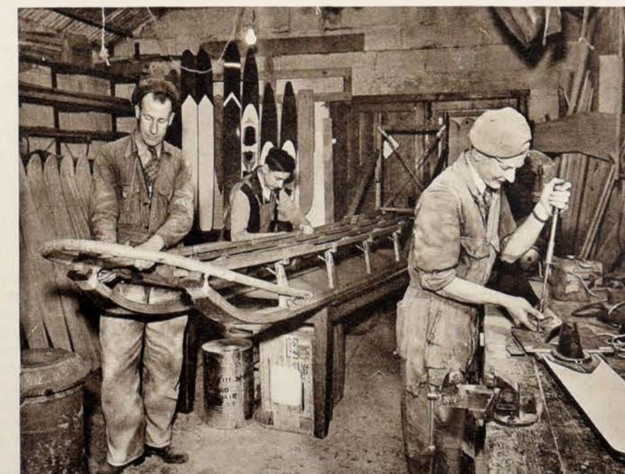
BUILDING SLEDGES FOR THE ANTARCTIC EXPEDITION: A workshop in a back street of Great Yarmouth, Norfolk, is the scene of the construction of sledges for the current Commonwealth Antarctic Expedition. Assembling a sledge in the picture are Mr. George Sheldrake (left) and Mr. Horace Sayers. On right of the picture Mr. Albert Griffith works on a water ski, one of the other products of the shop. Sledges and skis made by this tiny East Anglian firm are exported to countries all over the western world.
