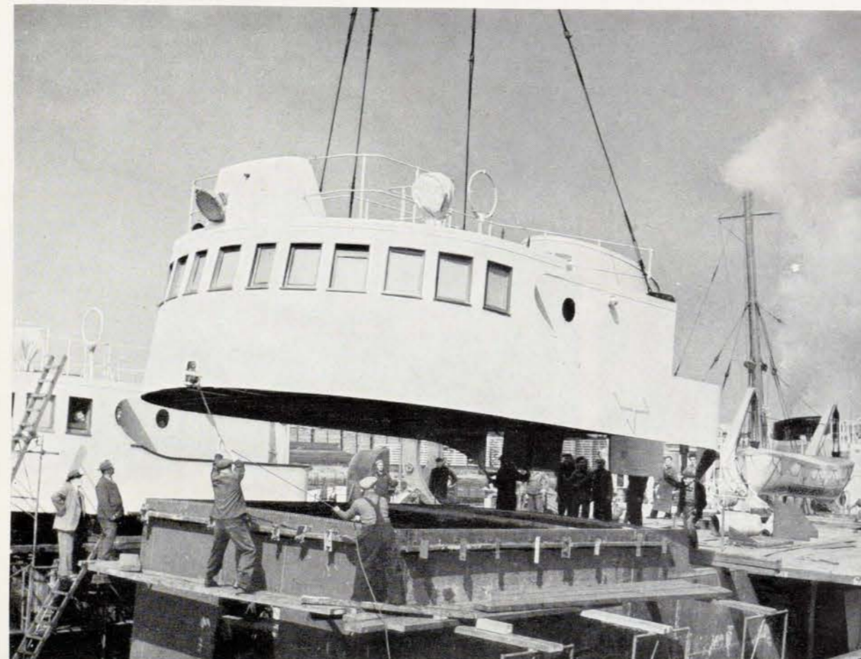
PART OF A SHIPBUILDING OPERATION WHICH IS CARRIED OUT WITH GREAT SPEED AND EFFICIENCY: A wheelhouse assembly is lowered on to the deck of the trawler. The Brooke Marine yard is so planned that it is able to complete a vessel in a remarkably short time. Present production of the 190-ft. trawlers results in a launching rate of one a month.
