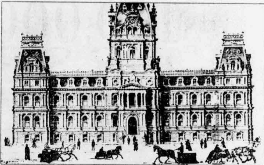
Montreal city hall in 1878: fire ravaged building in 1922, but stone walls remained secure.
