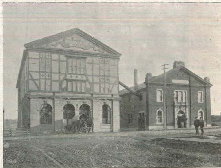
MILLS AT VICTORIA, B.C.
