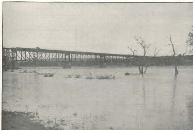
Great Northern Railway Bridge at Hawkesbury.
