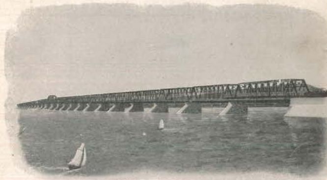
Victoria Jubilee Bridge over St. Lawrence River, Montreal
