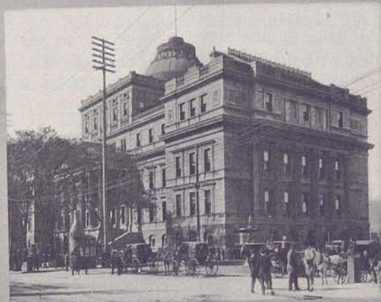
City Hall. Nelson Column. Court-House.
