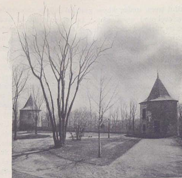
Towers in the Grounds of Montreal College, Sherbrooke Street, probably the Oldest Structures in Montreal, dating back some 250 years.
