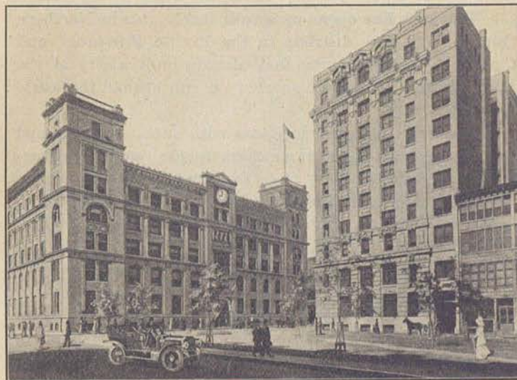
Offices of the Grand Trunk Railway System and of the Canadian Express Co., Montreal.
