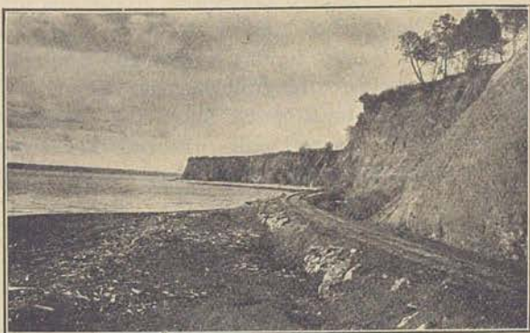
New Shore Line to Quebec—Canadian Northern Quebec Railway.
