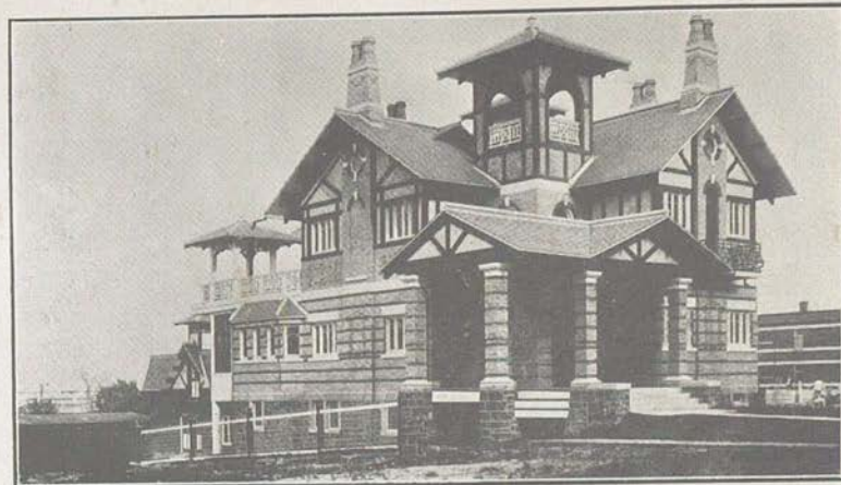
RESIDENCE OF MR. JOSEPH LAMOUREUX 143 St. Catherine Road, Outremont.
