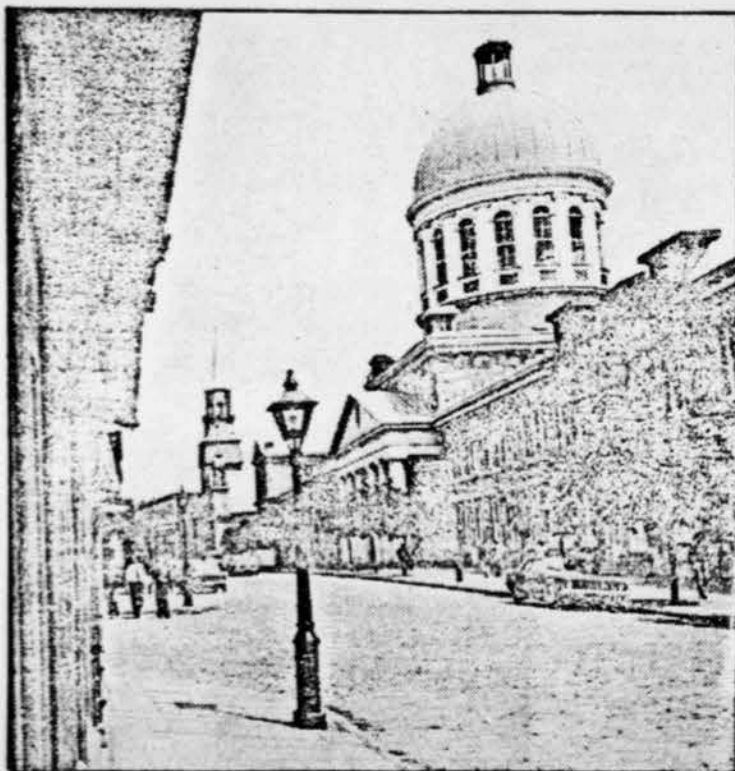
Older style: Coherent façades of Bonsecours Market.
