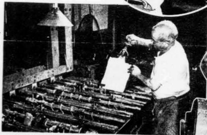
*Lowering a matrix into an electrolytic bath, a step in making electrotypes, facsimile plates used in printing.*
