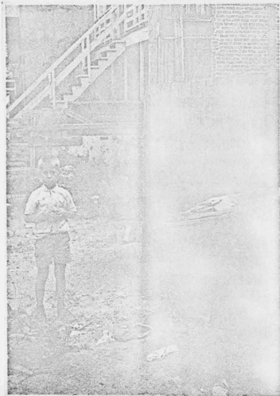
Hopefully, this lad will have a better backyard when reconstruction is completed.
