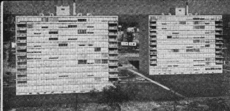
AFTER SIX YEARS OF TOIL, FOUR APARTMENTS ON FORMER SLUM SITE IN CHICAGO
