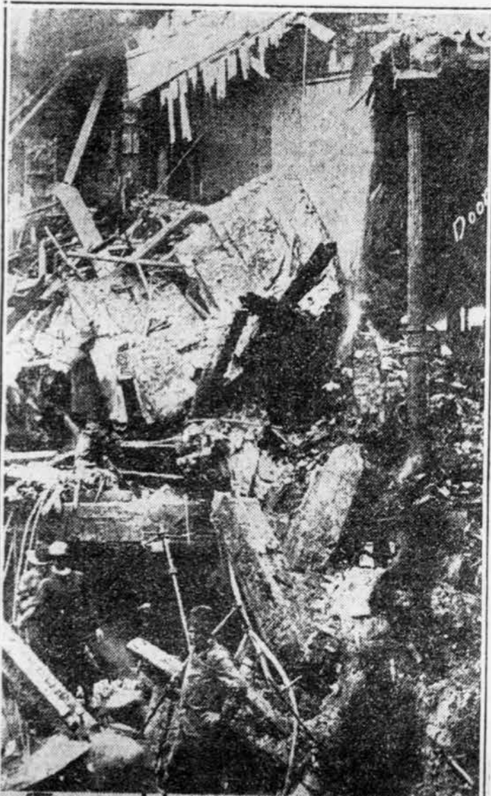
THE HERALD FIRE LOOKING FROM REAR EAST SHOWING DEPTH OF DEBRIS.
