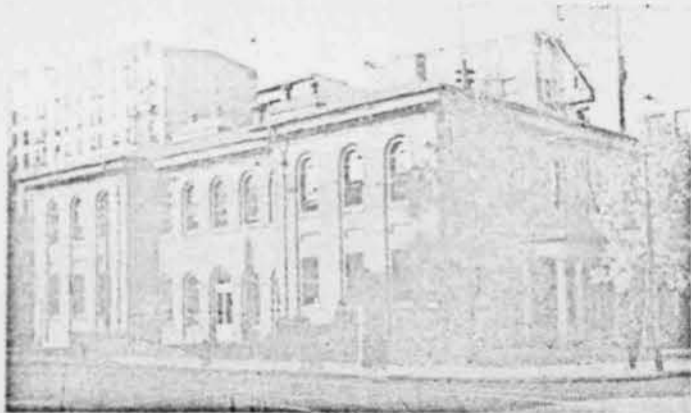
Now the Fraser Library, the school made its home here under its old name of Burnside Hall from 1854 to 1878.
